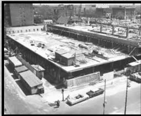
Construction in progress, April 16, 1964
